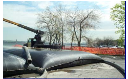
Geotextile tubes during passive dewatering.
